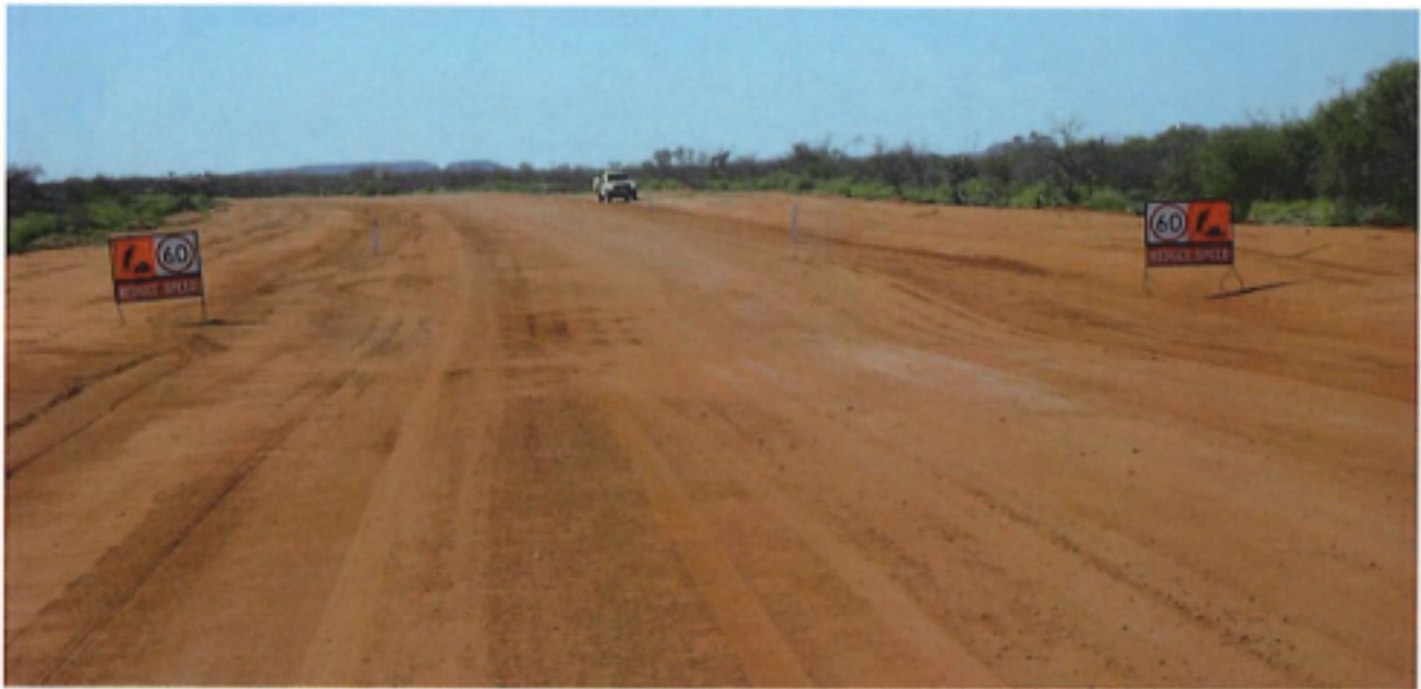
Ullawarra Rd S1k 8.4 - Completed.
