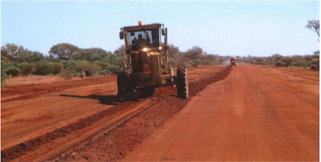
Cobra Mt Augustus Rd – Current works.
