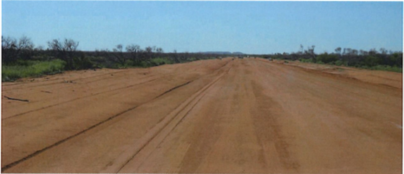
Ullawarra Rd S1k 8.00 - Completed.
