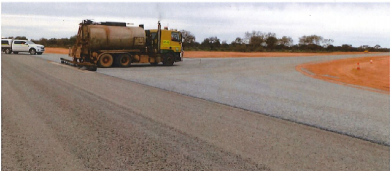
Dalgety Downs - Landor Rd SLK 76.90 - 005.JPG - Intersection Sealing.
