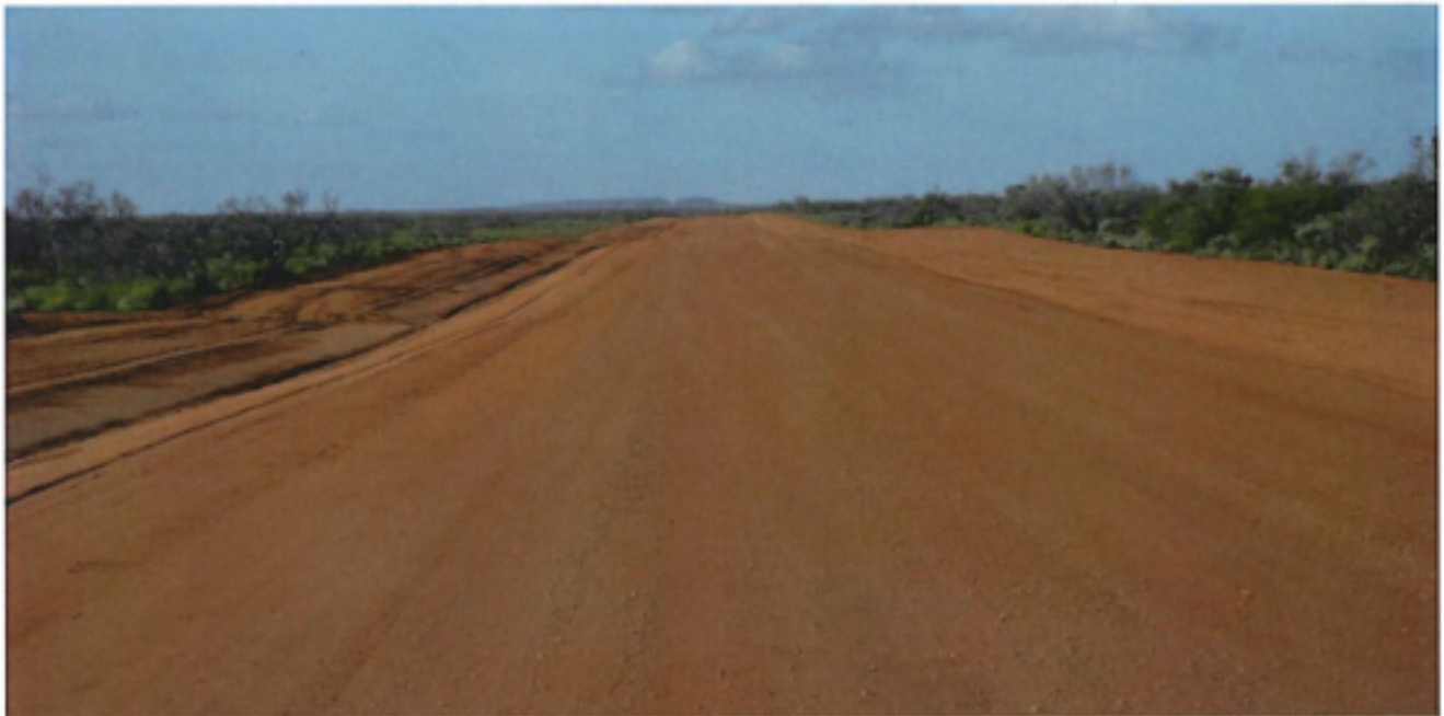
Ullawarra Rd Slk 6.7 - Completed.
