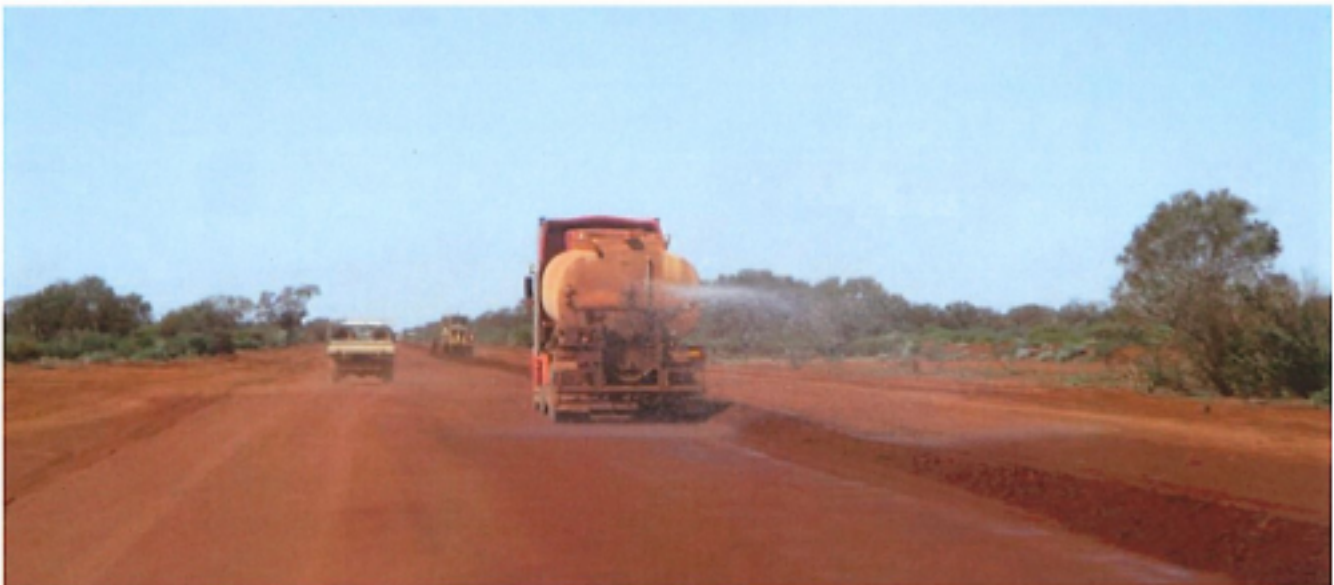
Cobra Mt Augustus Rd – Current works.
