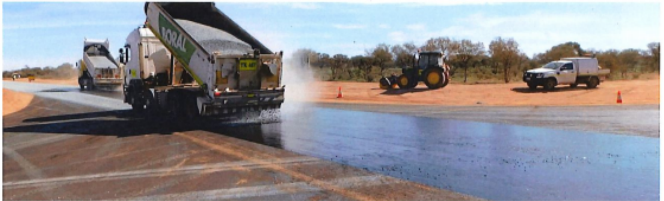
Dalgety Downs - Landor Rd SLK 76.90 - 003.JPG - Intersection Sealing.
