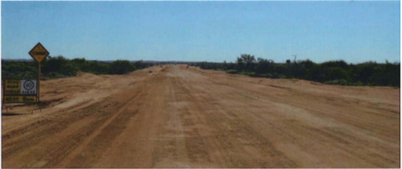
Ullawarra Rd Slk 3.5- Completed.
