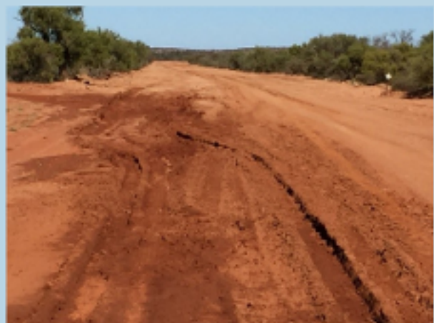
Landor Burringurrah Rd May 2016: driving on wet roads, estimated repair costs were $45,000.00
