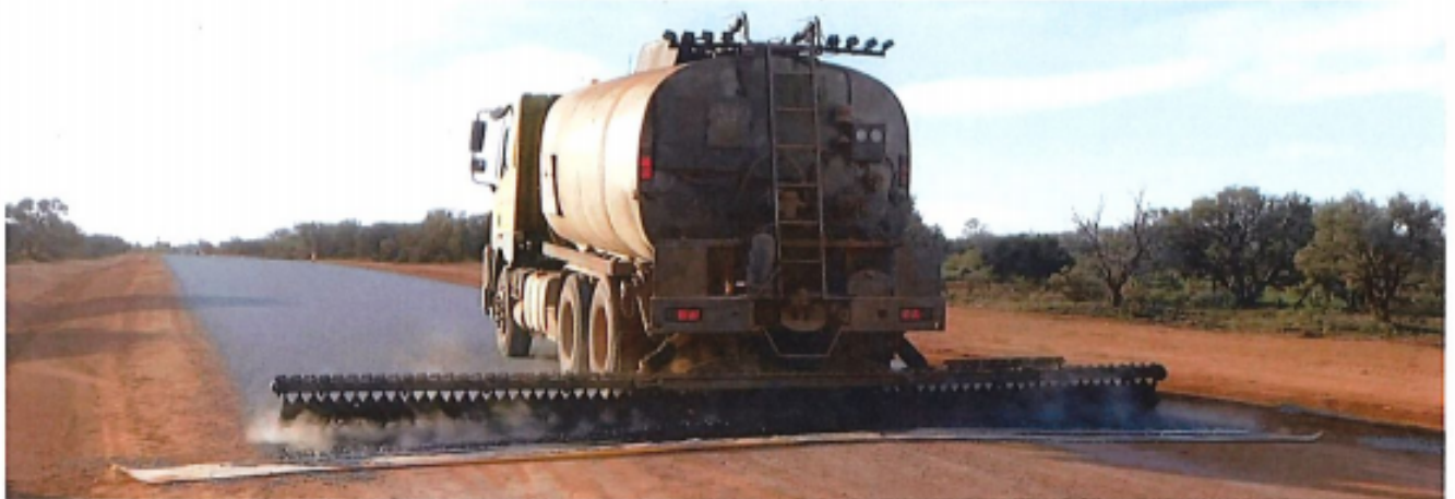
Dalgety Downs - Landor Rd SLK 76.90 - 004.JPG - Intersection Sealing.
