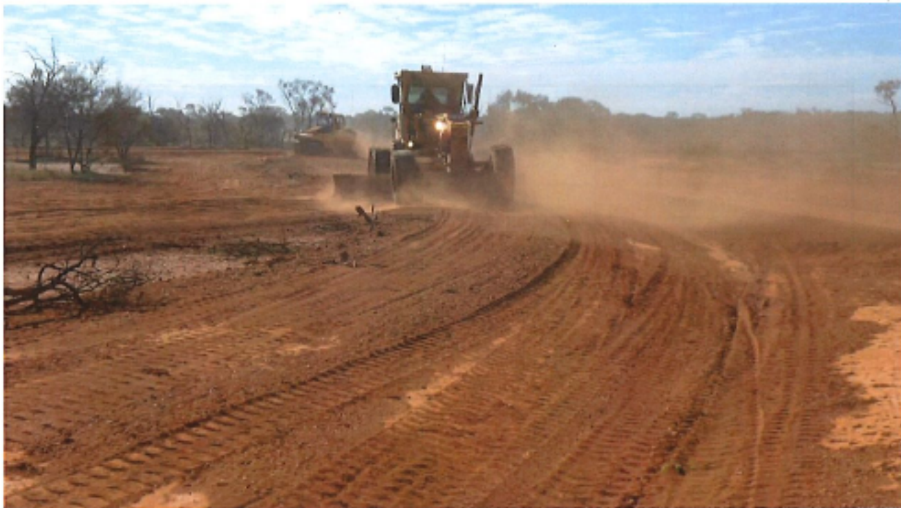
Ullawarra Road – Current Works
