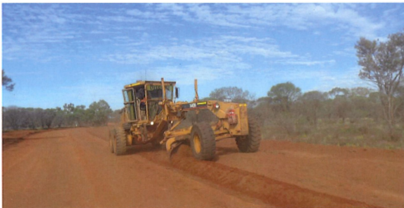
Ullawarra Road – Current Works
