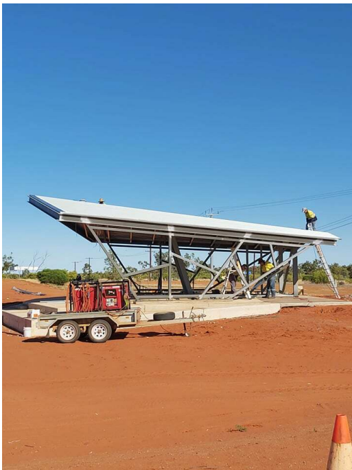
The roof is installed on the Ampitheatre at the Visitor Stop
