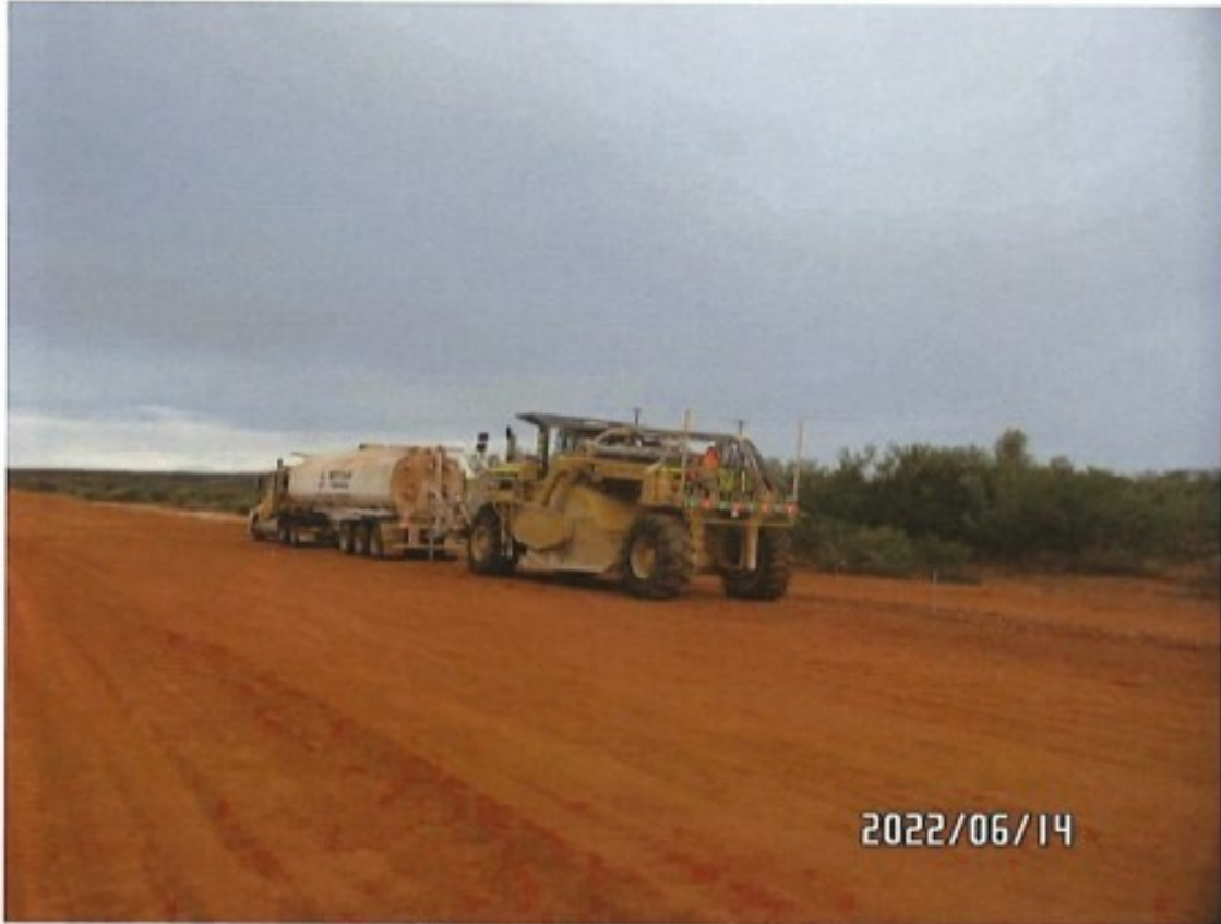
Carnarvon Mullewa Rd – Floodway stabilisation works.
