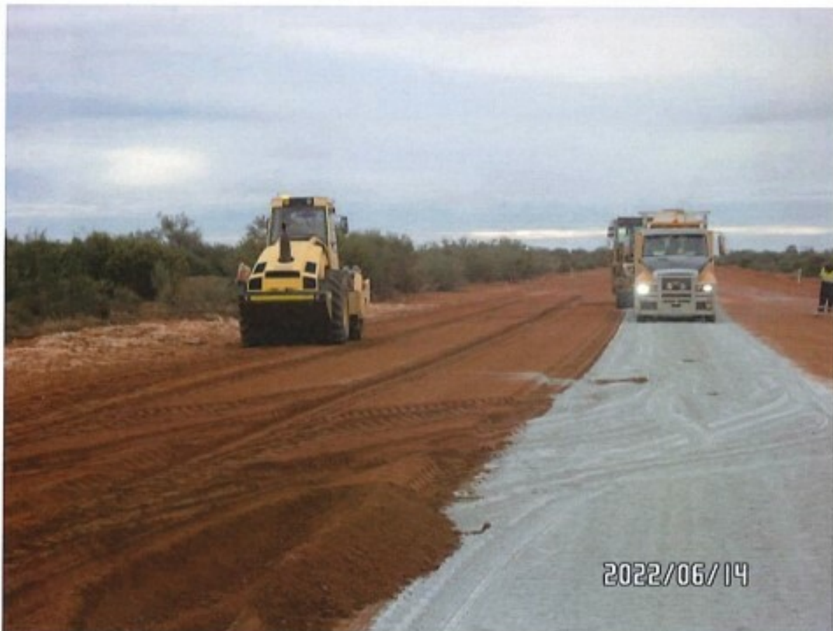
Carnarvon Mullewa Rd – Floodway Stabilisation works
