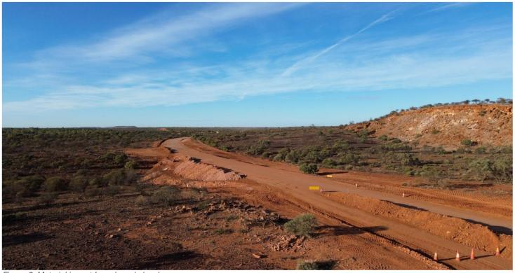
Figure 2: Material import for subgrade level
