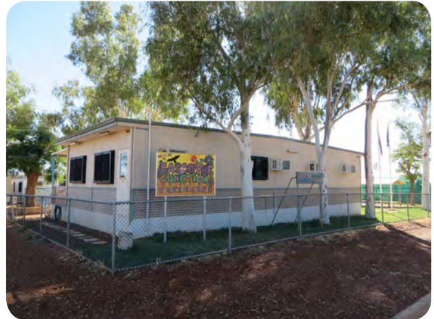
Gascoyne Junction Remote Community School
