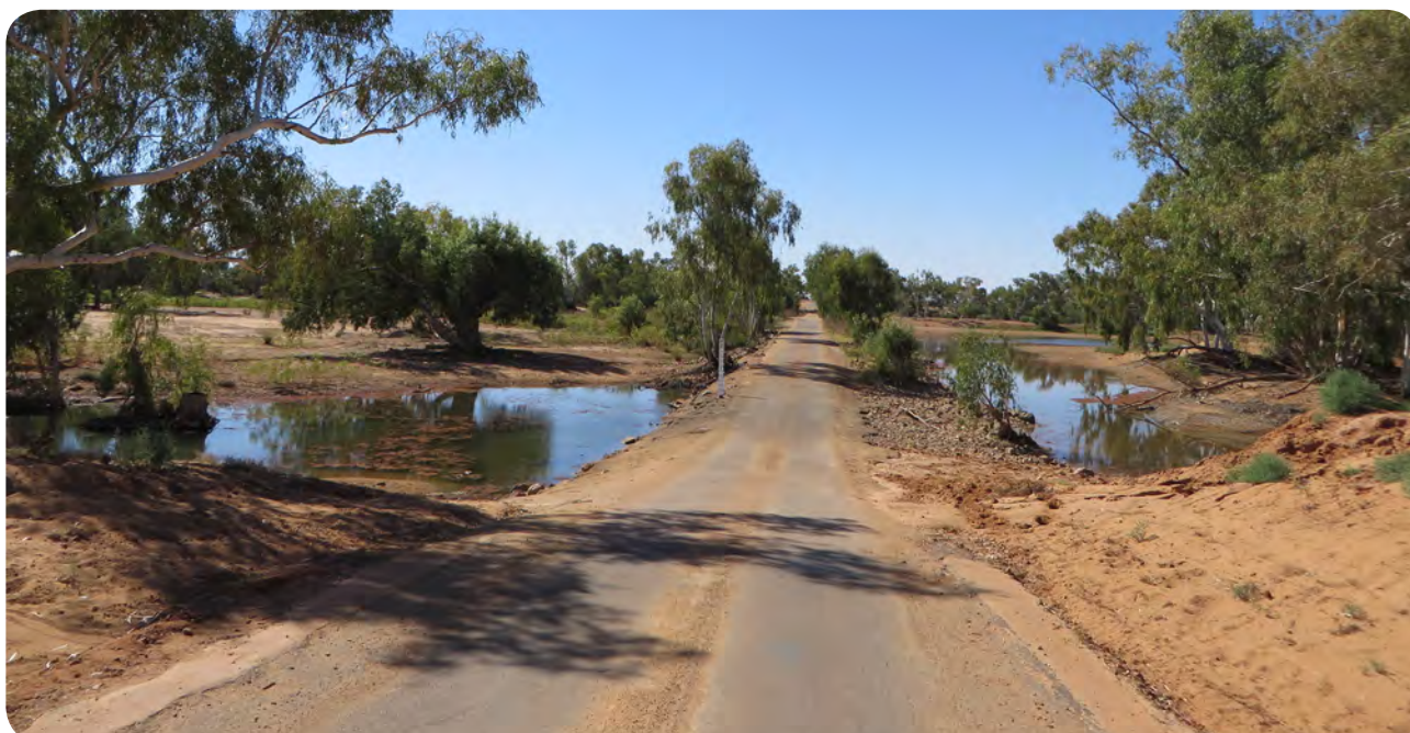
Existing Gascoyne River crossing
