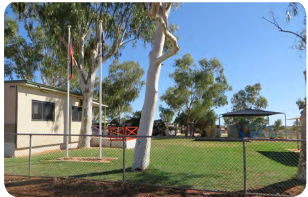
Gascoyne Junction Remote Community School
