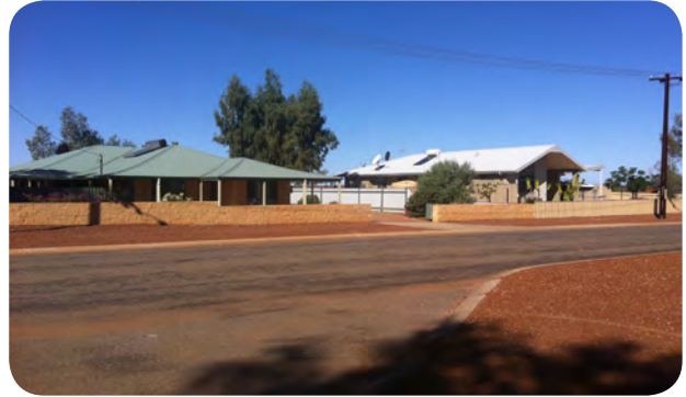
Gascoyne Junction housing
