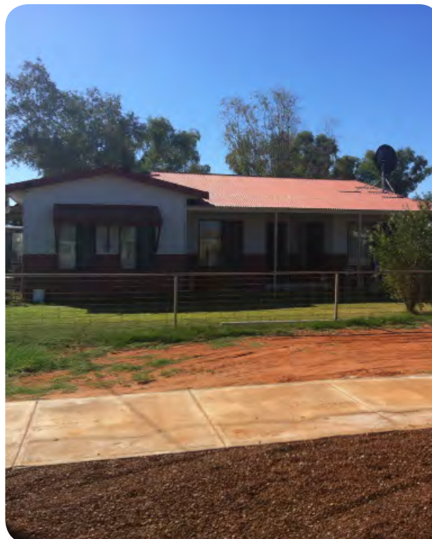
Gascoyne Junction housing
