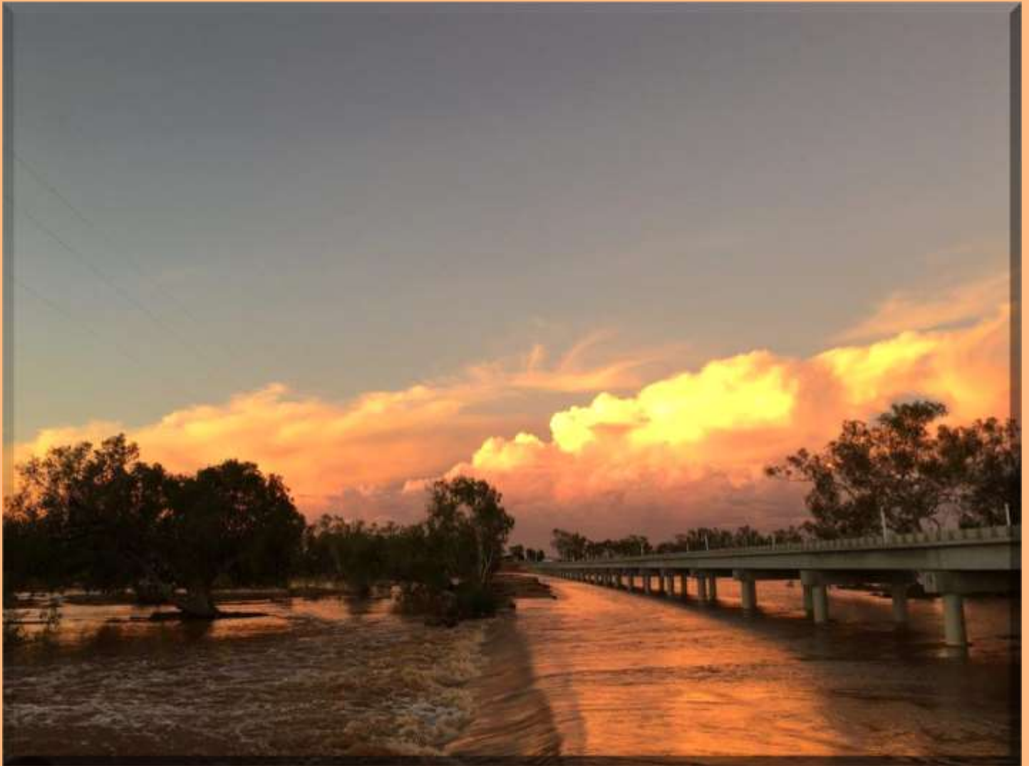
First River flow for 2017 - under the newly built Killili Bridge at Gascoyne Junction river crossing.
