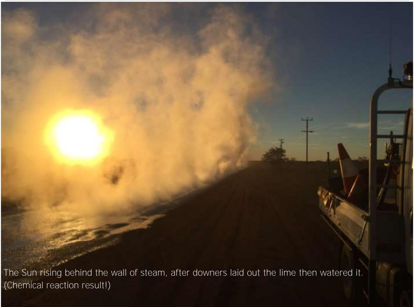
The Sun rising behind the wall of steam, after downers laid out the lime then watered it. (Chemical reaction result!)
