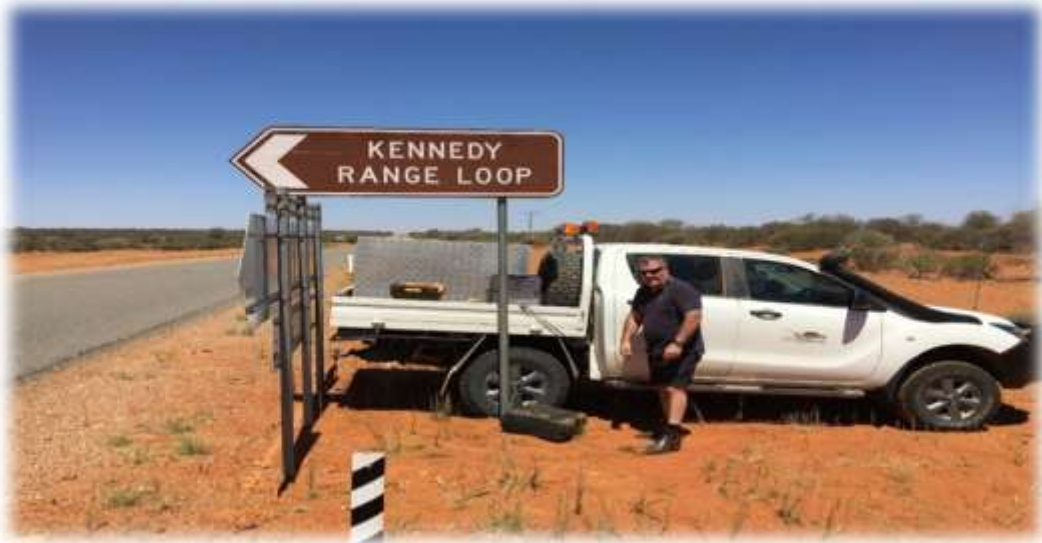
Kennedy Loop sign installation
