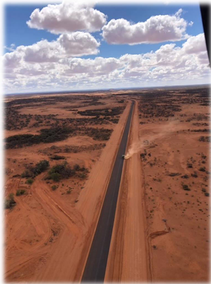
(New bitumen on Carnarvon Mullewa Road)
